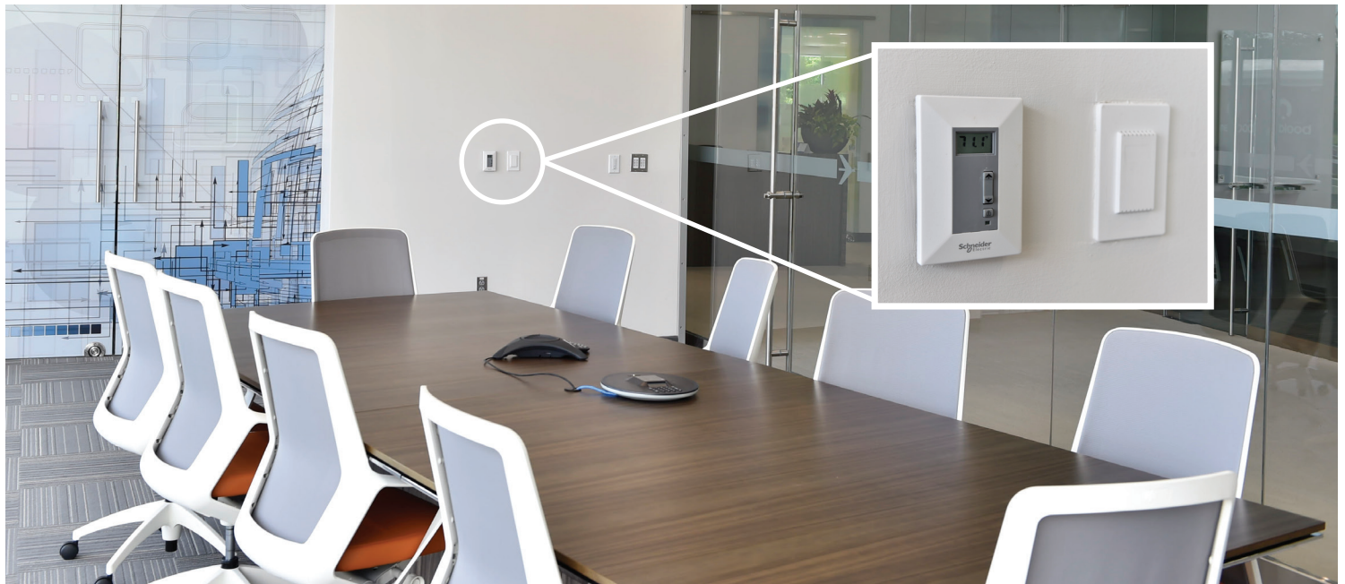
A DCV sensor (on the right) can easily be added to your existing Heating Ventilation Air-Conditioning (HVAC) system and is typically located next to a thermostat.
