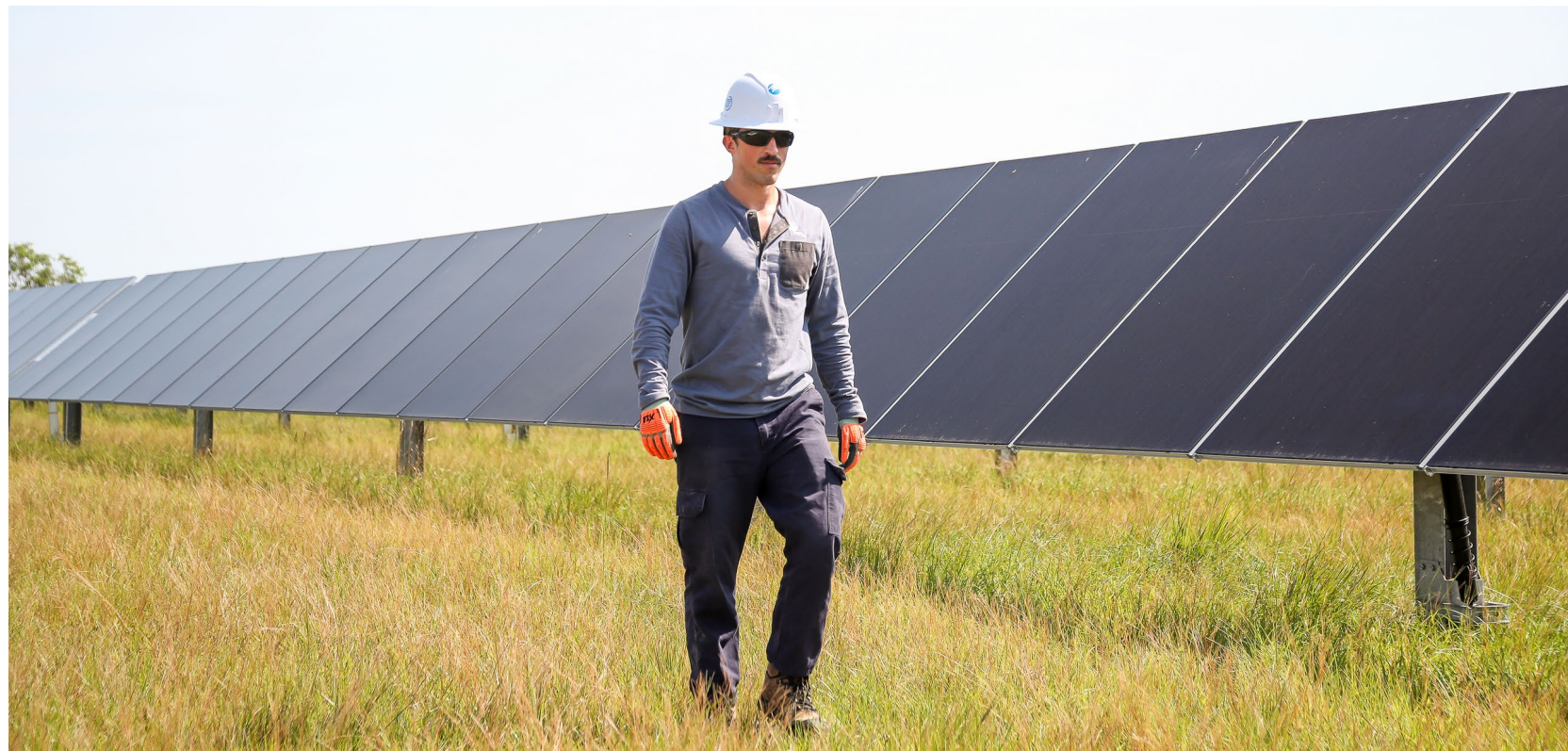
Employee Gavin Hunt walks among the solar panels at the Cavendish Solar Energy Center in Okeechobee, Fla.
