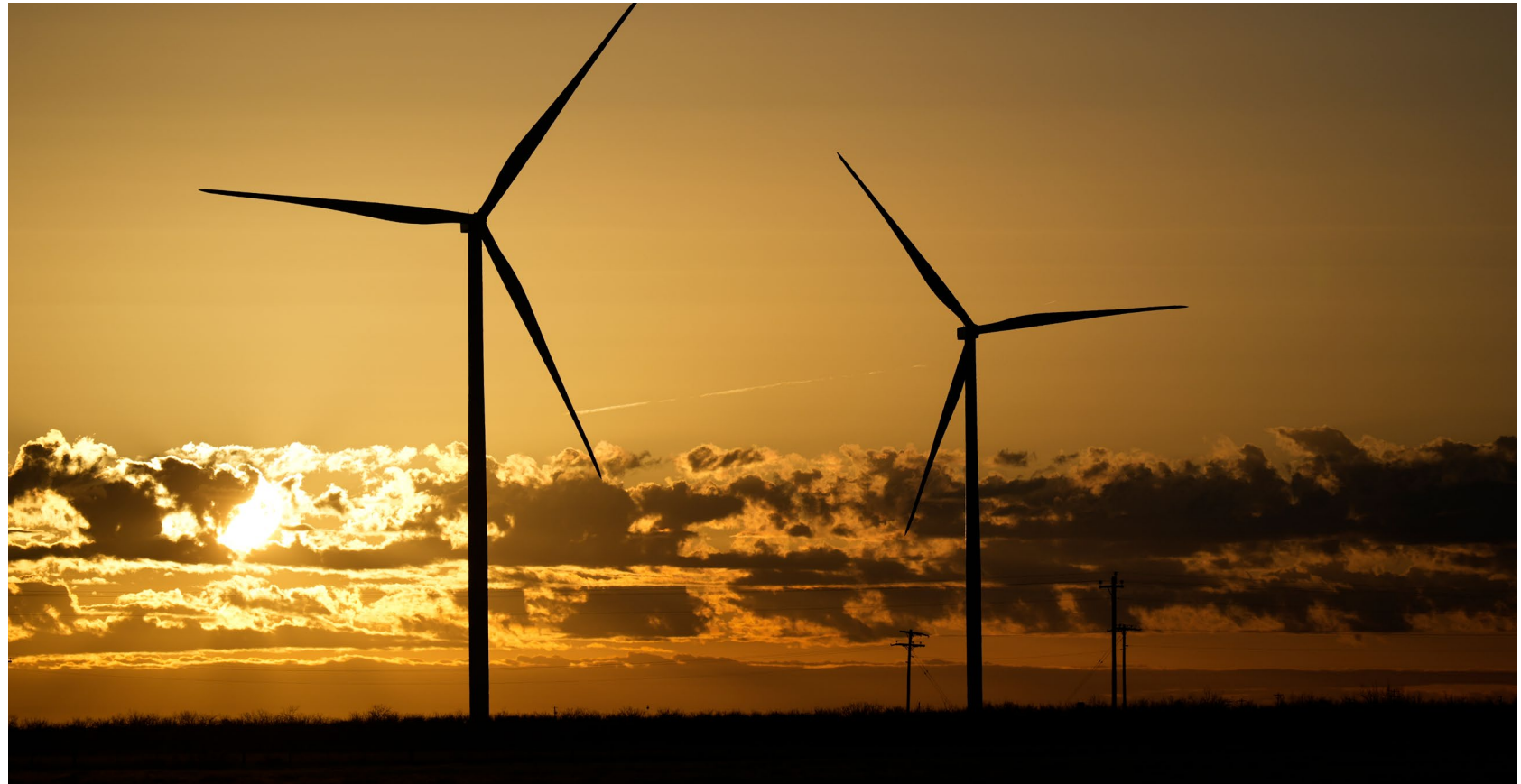
Lacy Creek Wind Energy Center in Glasscock and Sterling counties, Texas.
