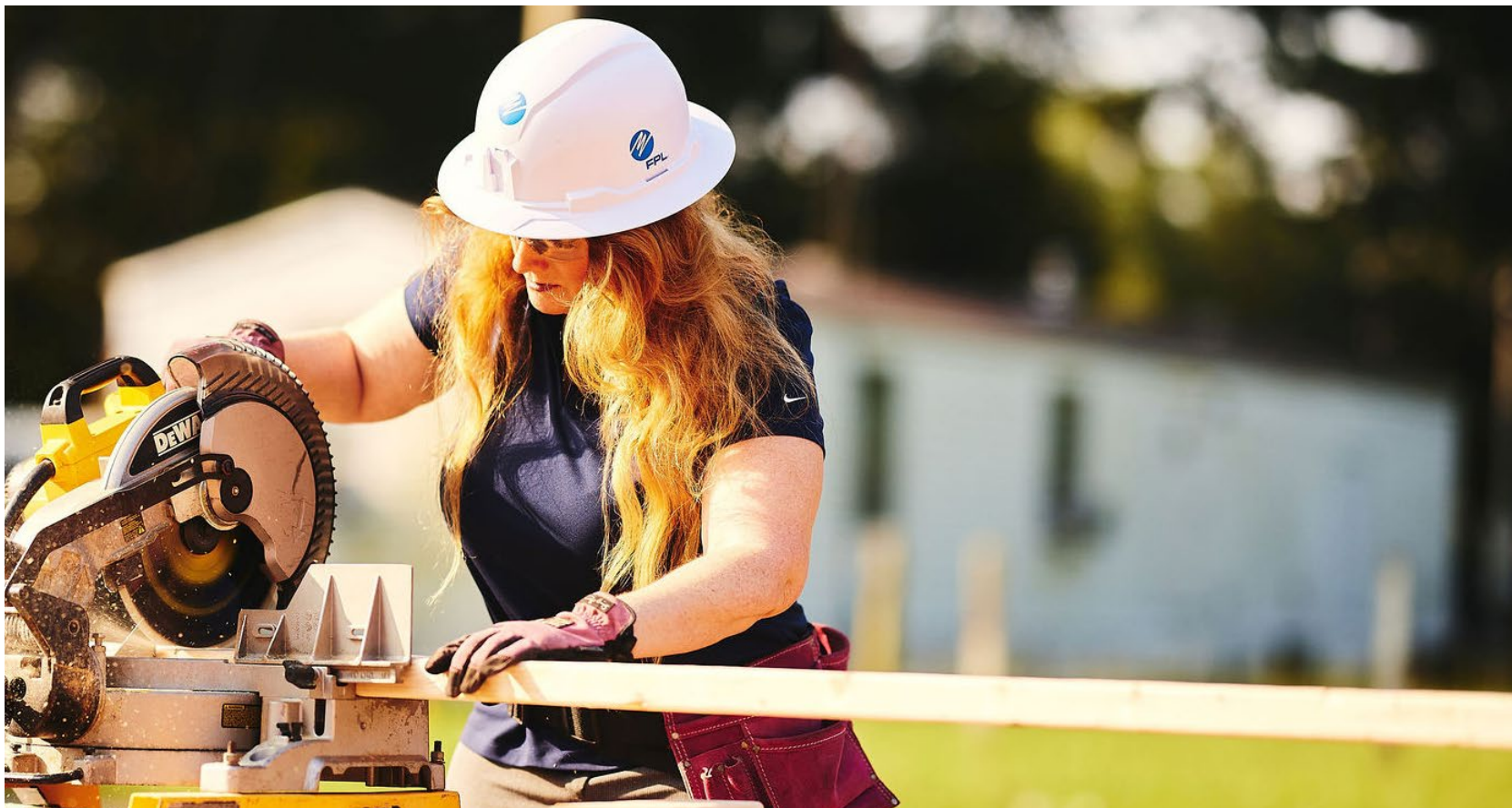
Employee Heather Madison uses a saw while volunteering at Pensacola Habitat for Humanity, one of many organizations supported by the NextEra Energy Foundation.
