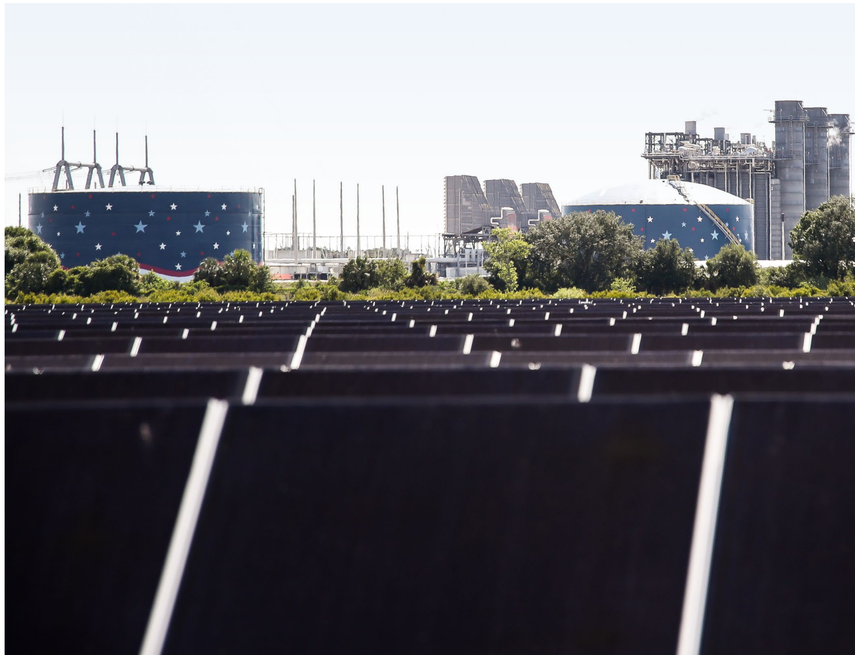
Cavendish Solar Energy Center in Okeechobee, Fla.
