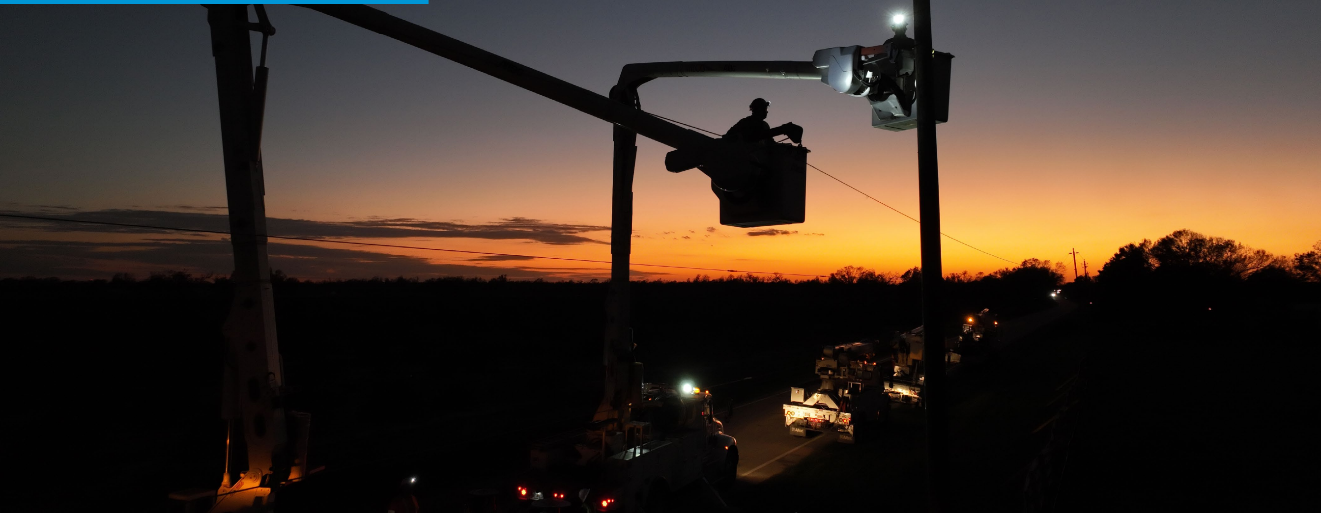
Crews work to restore power in Arcadia, Fla., following Hurricane Ian.
