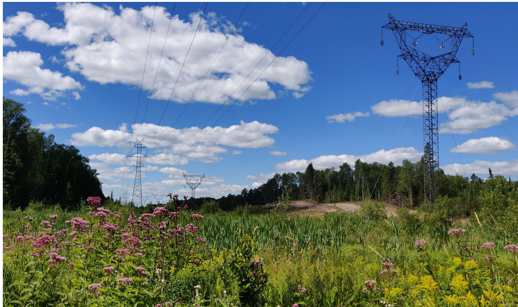
East-West Tie transmission line in Ontario, Canada.
