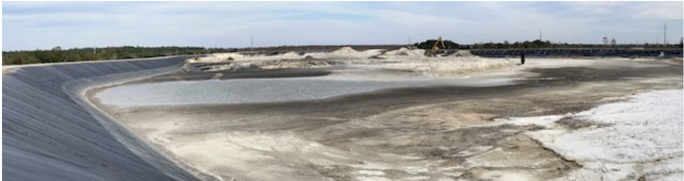
Figure 1: Panorama Photograph at Time of Inspection – GCEC Gypsum Storage Area
