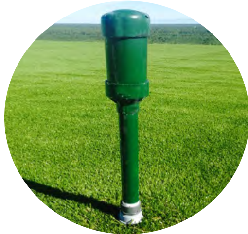
After valve is installed.
