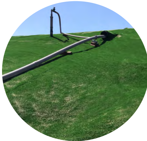
ClosureTurf integrates easily with traditional gas systems.
