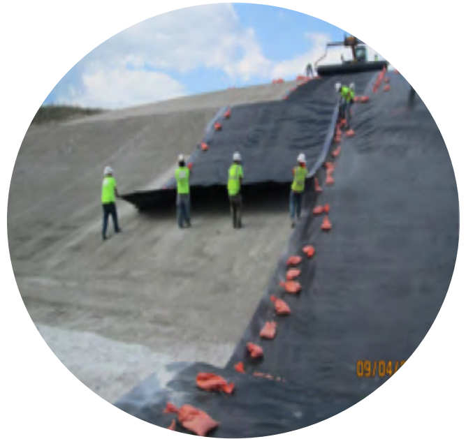
Workers manually unroll the membrane down the slope.
