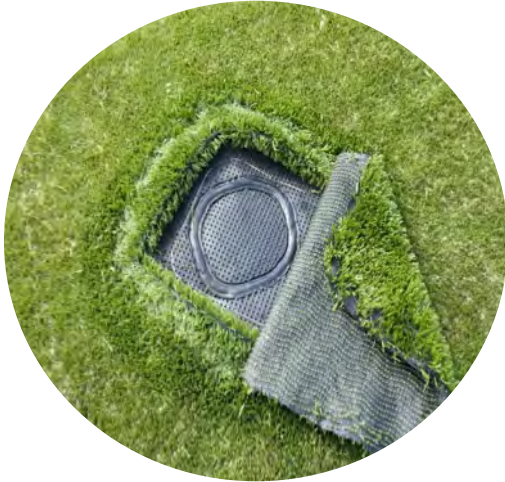
Before valve is installed.
