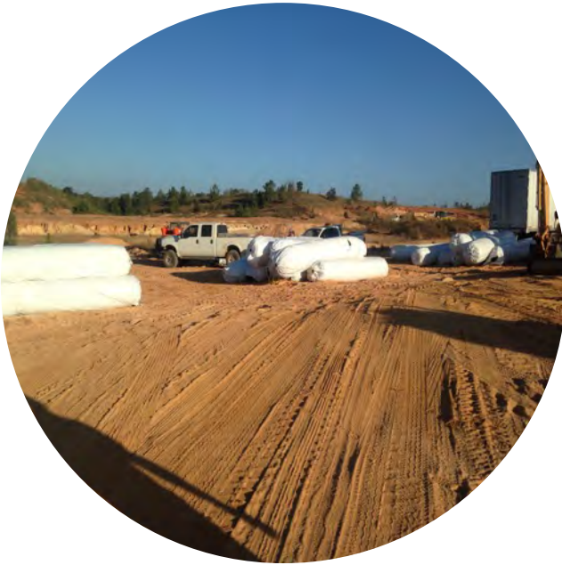
Geomembrane arrives on site in rolls.
