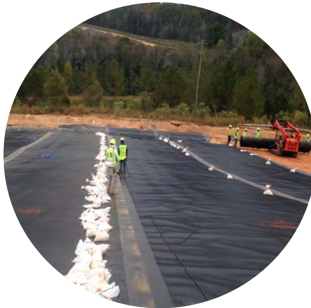
Geomembrane seams are heat welded together.
