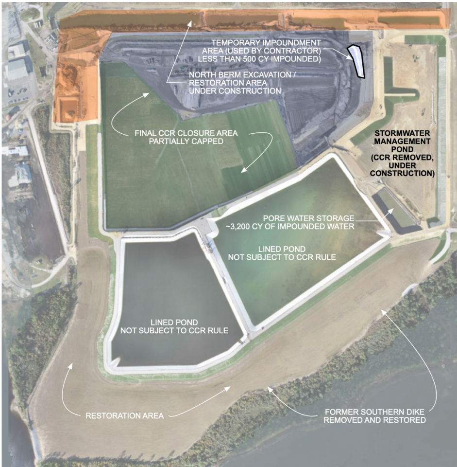
Figure 1: Aerial Image of Plant Smith Impoundment dated December 6, 2023
