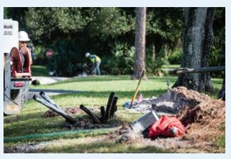
directional boring or horizontal directional drilling, installs underground piping to safely place our electric cable to connect power to your home or business. Unlike open trenching, directional boring allows FPL to install underground equipment while minimizing impact to trees and other vegetation on your property. The underground facilities will be installed 36 inches to 48 inches below the surface, or deeper, if necessary, to avoid tree roots.
